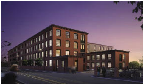
The Grant Mill Building - Providence, RI
